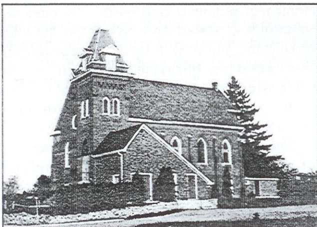
Copetown Church - Renovations - 1968
